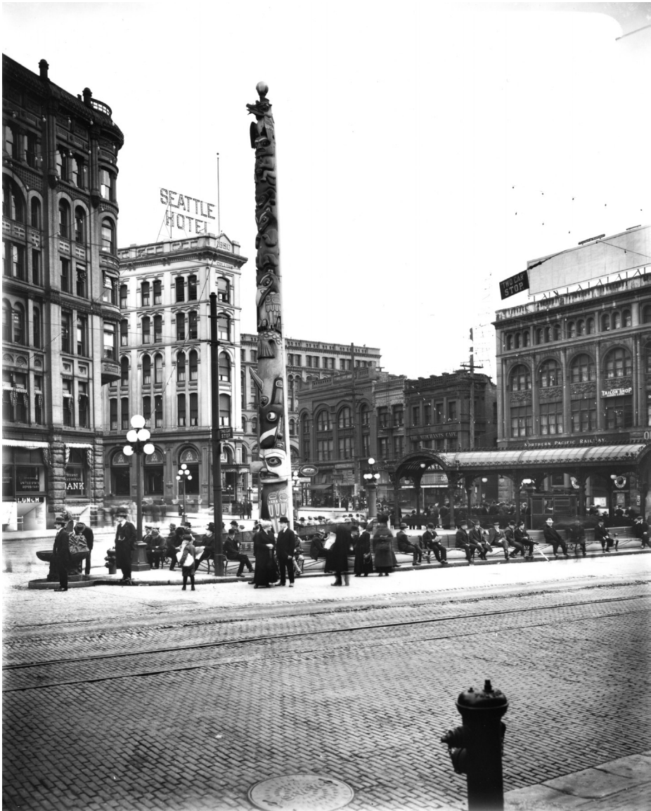
Pioneer Square totem pole and pergola, Seattle, n.d. Photographer: Calvin F. Todd.
