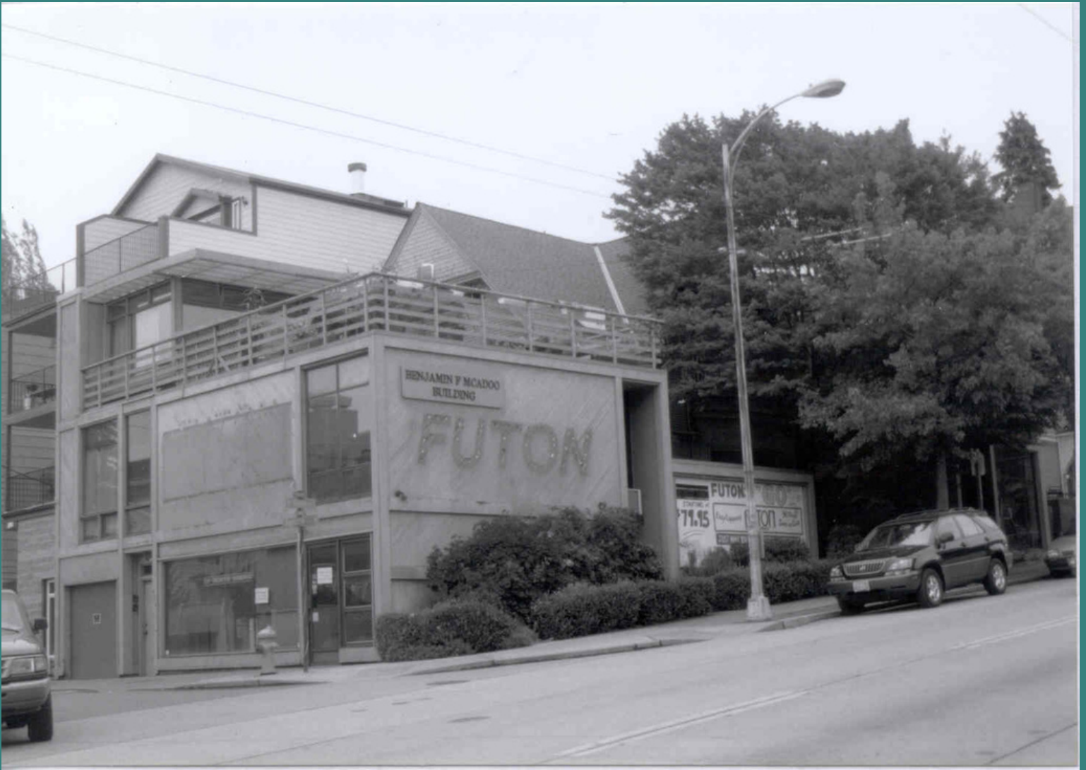
Benjamin F. McAdoo Office, designed by McAdoo. Image taken August, 2001. Seattle Historical Sites.
